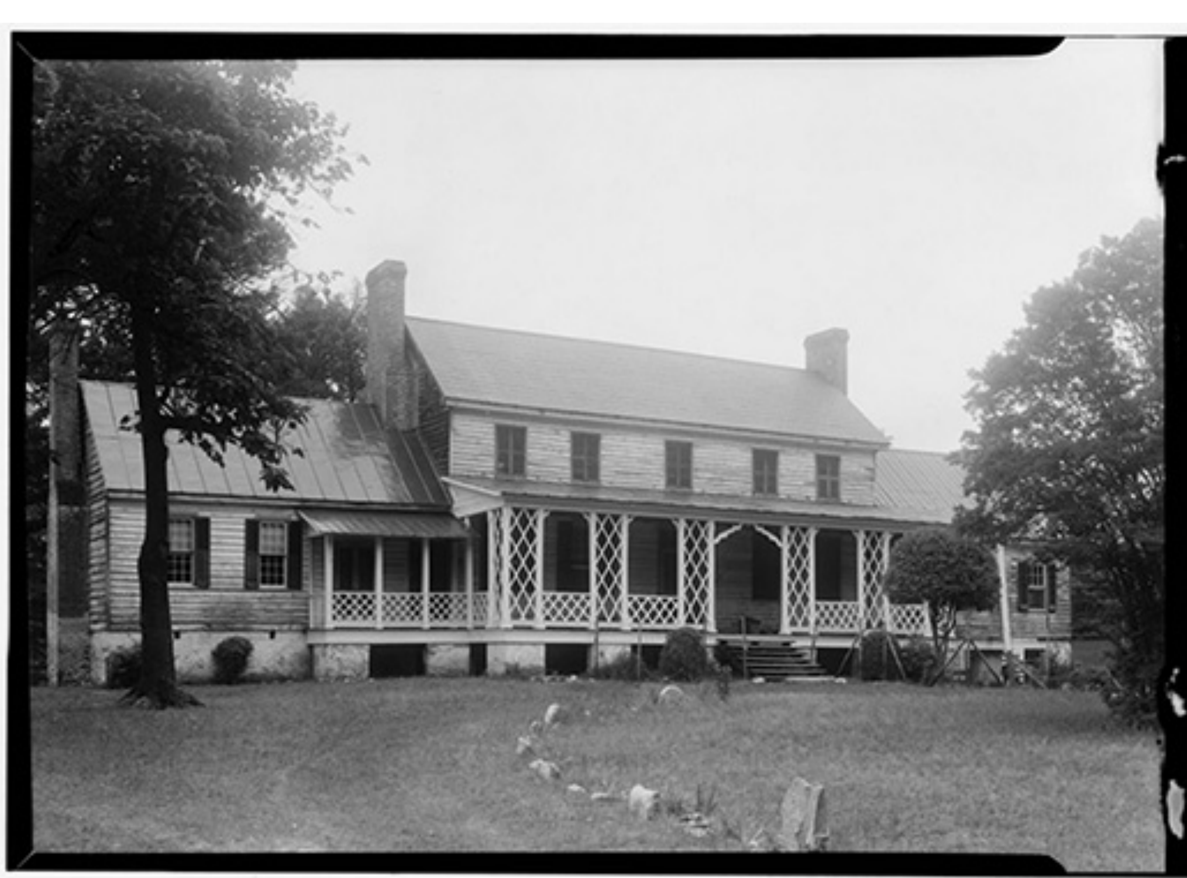
Fonthill, State Route 631 vicinity, Champlain, Essex County, VA . Documentation compiled after 1933. Historic American Buildings Survey/Historic American Engineering Record/Historic American Landscapes Survey . Prints & Photographs Division
