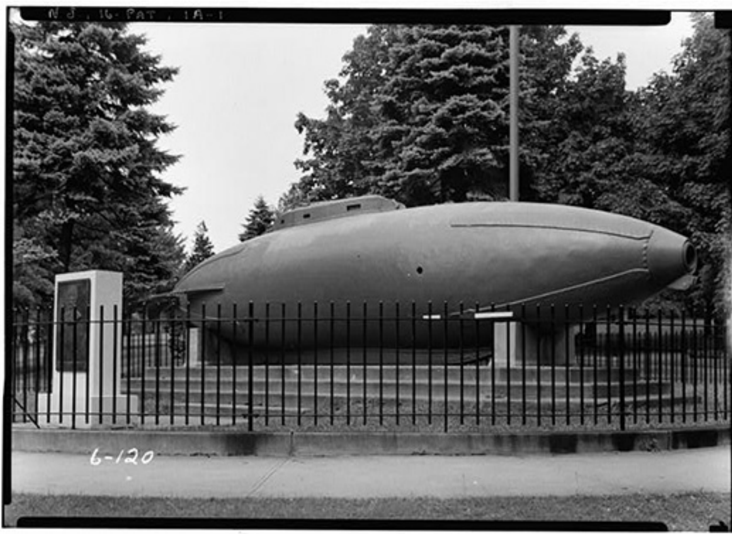
The Holland Submarine, Paterson, Passaic County, NJ. Nathaniel R. Ewan, photographer, July 17, 1936. Historic American Buildings Survey/Historic American Engineering Record/Historic American Landscapes Survey . Prints & Photographs Division
